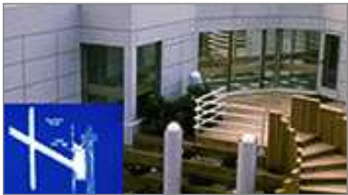
建筑外装饰中铝制面板粘贴于金属框架 The aluminum panel is attached to the metal frame in the exterior decoration
